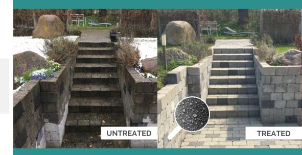
Super Hydrophobic Self-Cleaning
